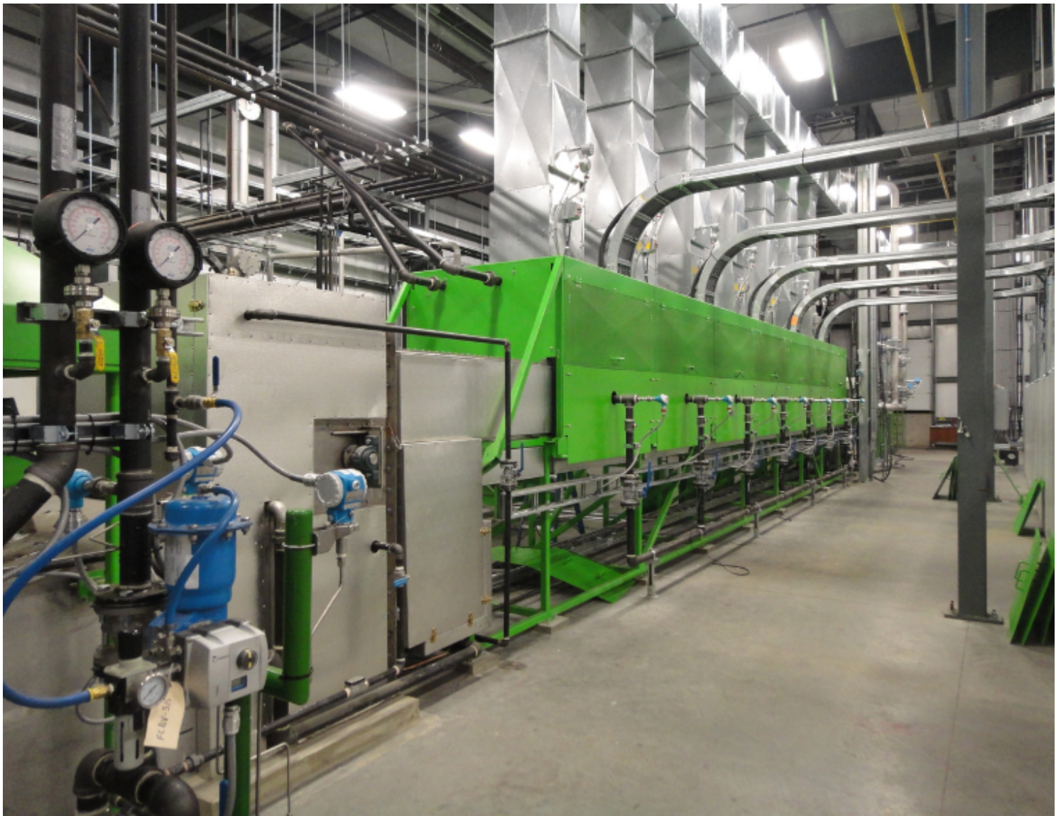
A processing tunnel for carbon black recycling at Environmental Waste International. Photo Environmental Waste International
